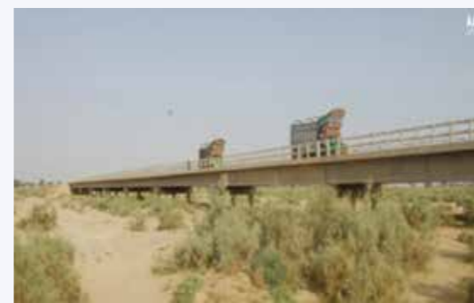
Ghankara Bridge Govt. Of Sindh
