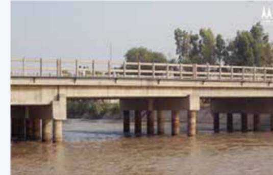
KB Bridge, Govt. Of Sindh
