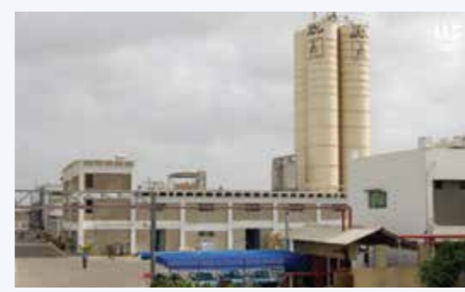
Pak Petro Chemical Warehouse, Karachi
