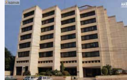
Sui Southern Gas Company, Lahore
