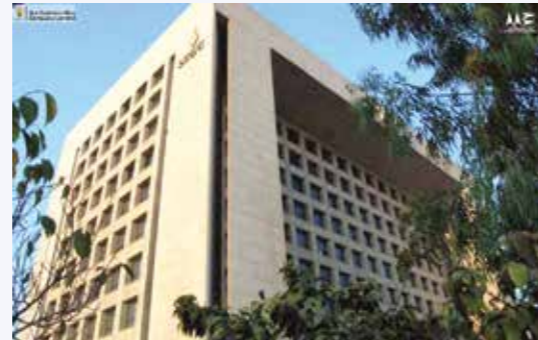
Sui Southern Gas Company, Karachi
