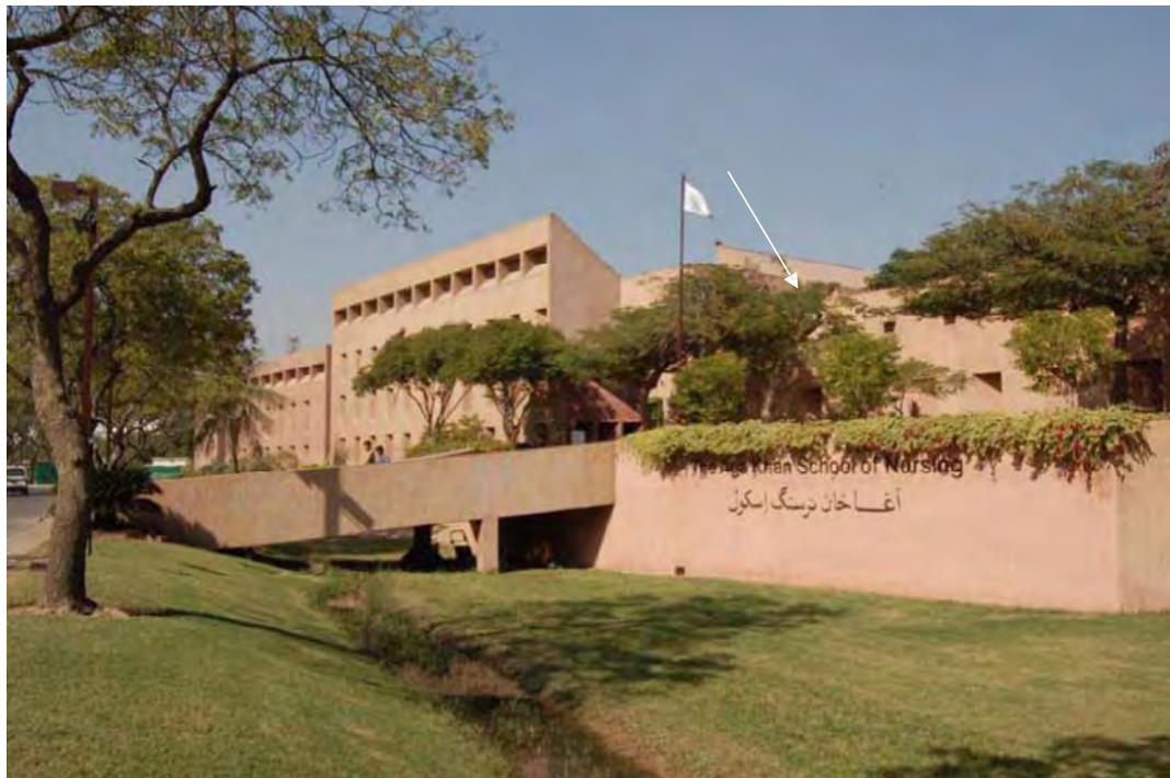
One million square ft AKU, Hospital at Karachi Architect: M/s Payette Associates, Boston, USA
