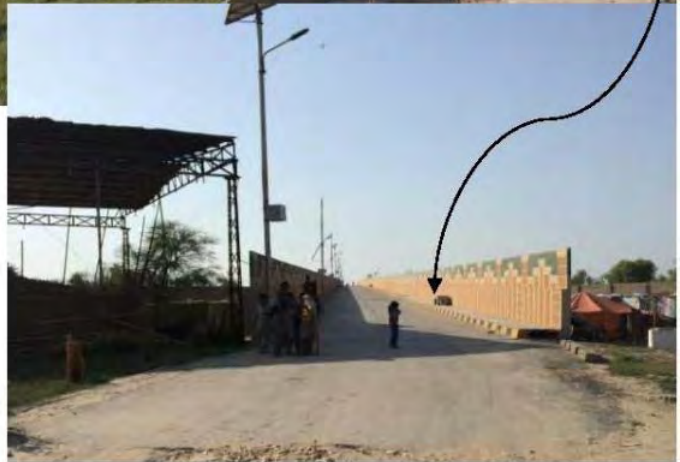
Bridge at Ghotki Dist, Province of Sindh Client: Govt. of Sindh
