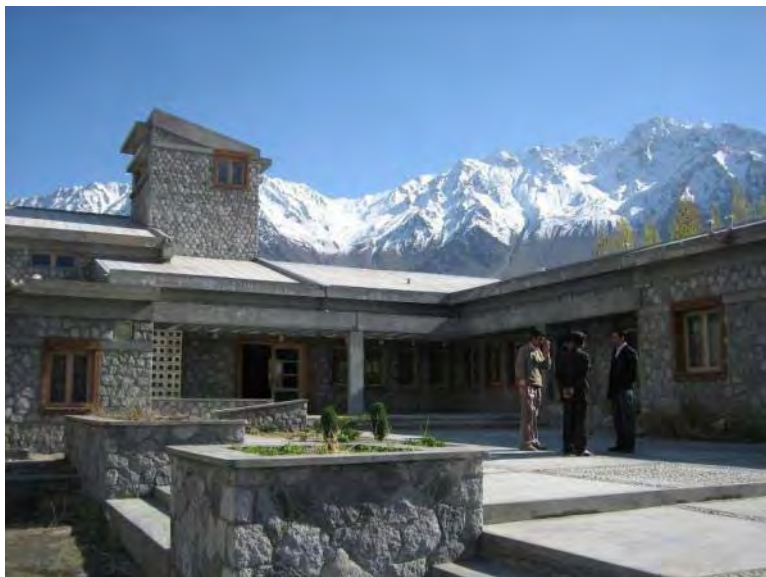
AKESP School at Gakoch, Gilgit Architects: M/s The Architects
