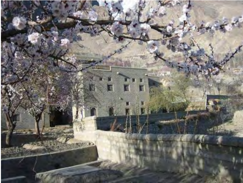
Girls Academy at Hunza located in high seismic zone in Pakistan Architect: Didier Leford of Paris France
