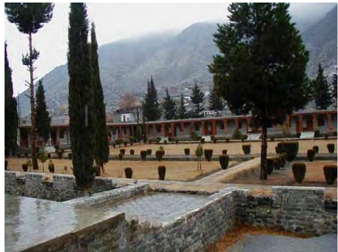
Seismic Strengthening of Shah Karim Hostel, Gilgit, Pakistan.
