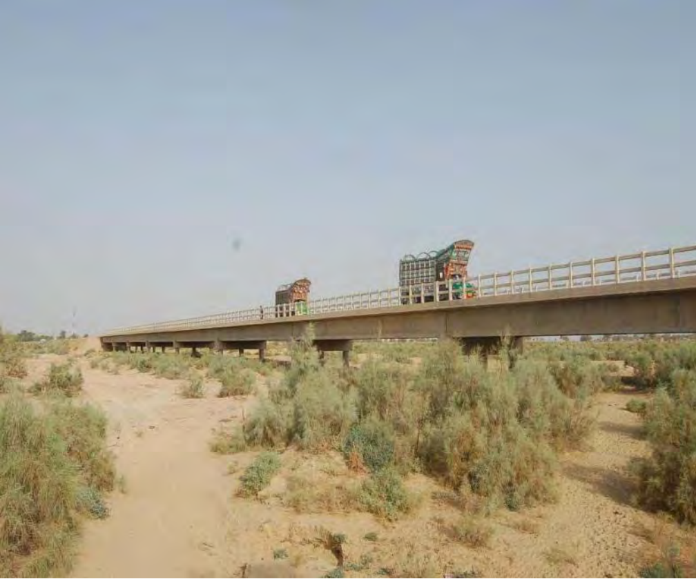
Ghankara Bridge Client: Govt. of Sindh
