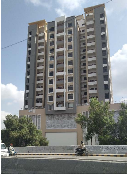
18-Storey A.T. One Tower at Karachi Architect: M/s Combined Associate, Karachi.
