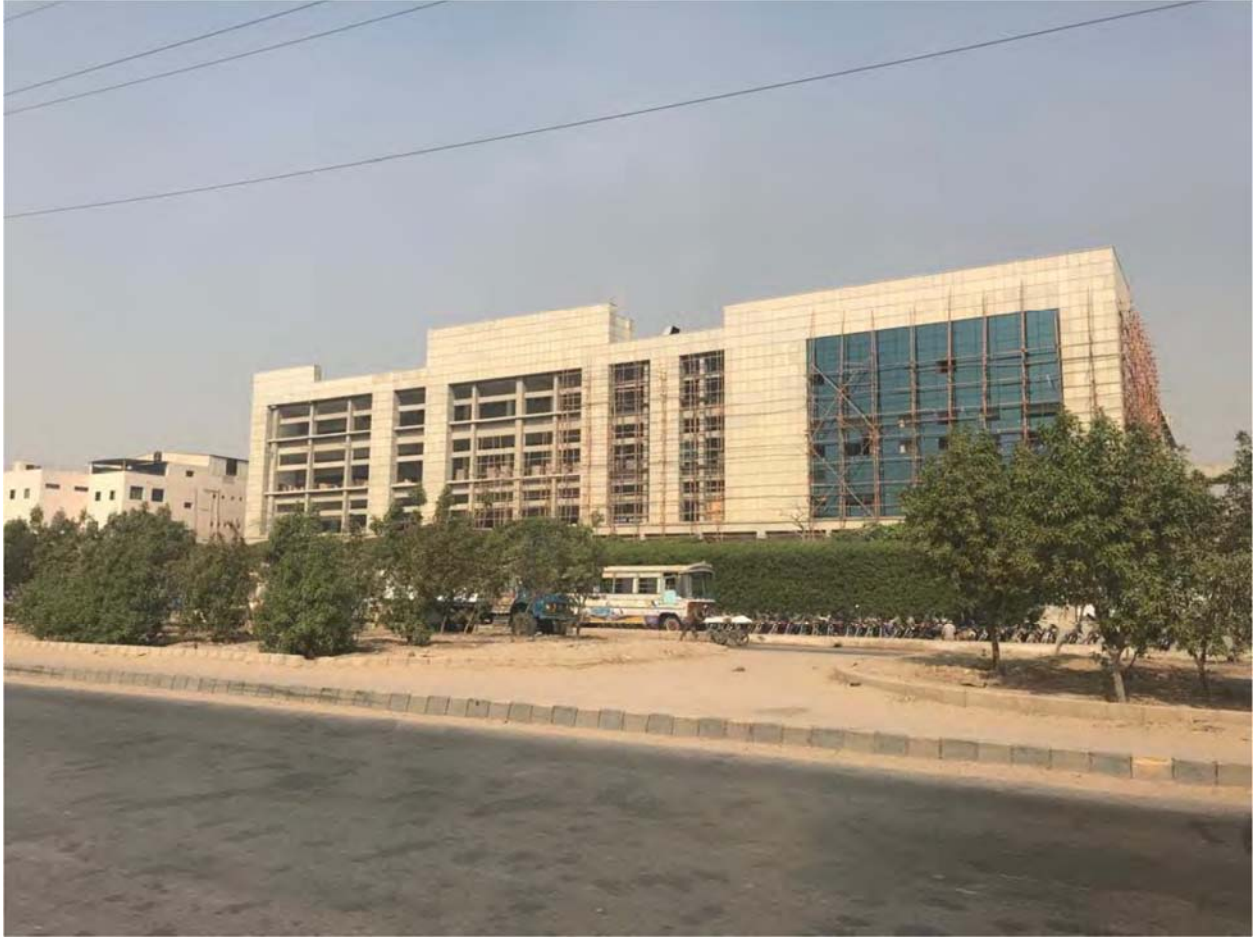
Artistic Denim Mills Building No: 3 Architect: Kareem Thobani
