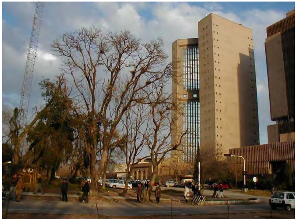
20 Storied HBL , Islamabad Architect: M/s AHED Associates
