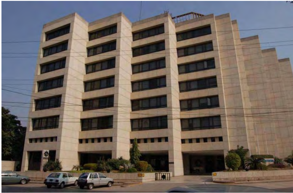
11 Storied Fair Faced Concrete Building, SNGPL Head Office , Lahore Architect: M/s Habib Fida Ali
