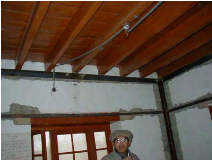
Strengthening of old pre-cast building at Khorog, Tajikistan; the building is used as temporary campus of UCA
