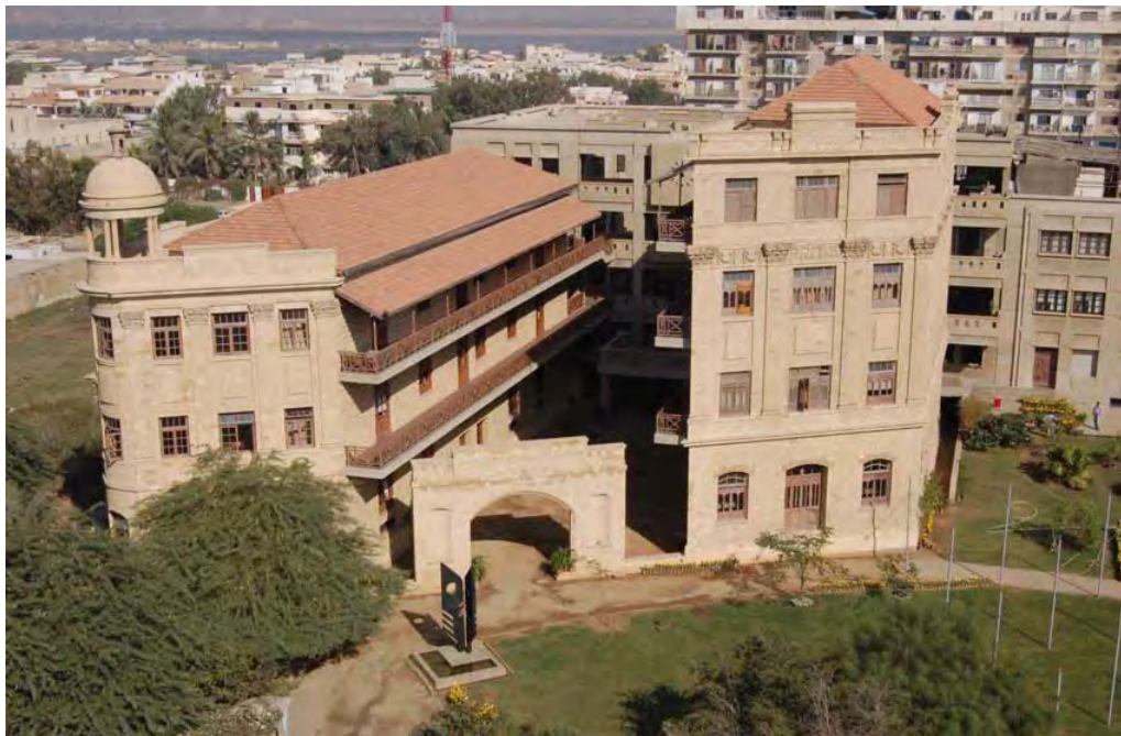
Indus Valley School of Arts and Architecture at Clifton, Karachi. This 100 years old building was stone by stone relocated, from Marry Weather Tower to Clifton.
